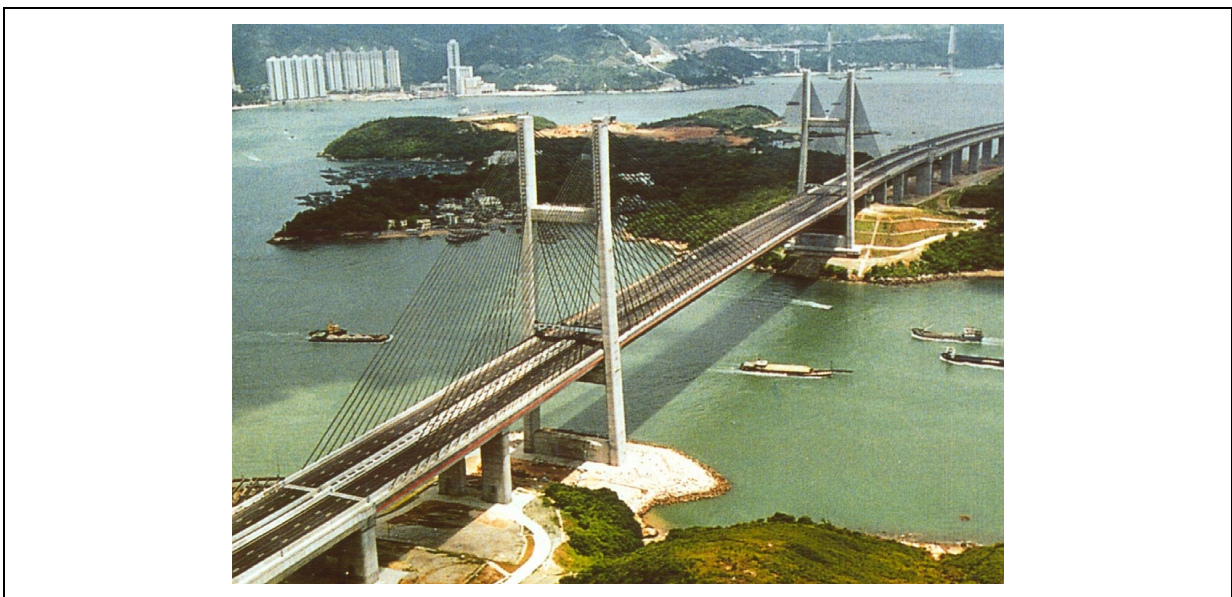
Figure 10 The Kap Shui Mun Bridge at Hong Kong
