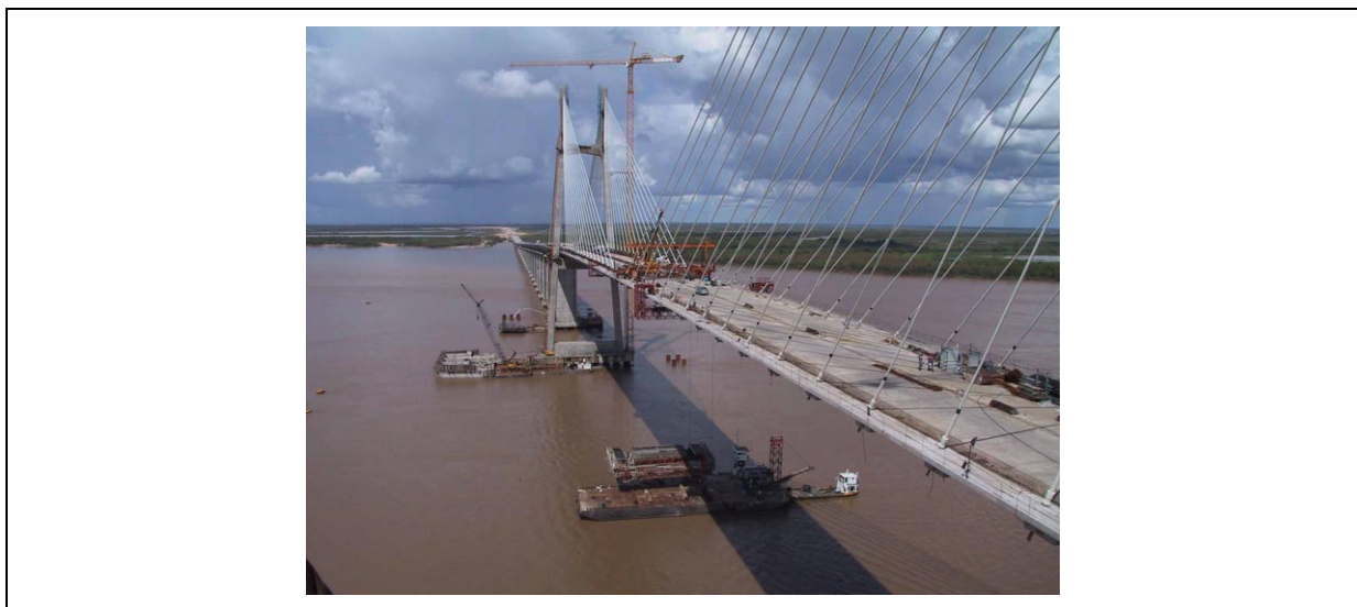
Figure 11 Cable-stayed bridge across the Paraná River between Rosario and Victoria, Argentina
