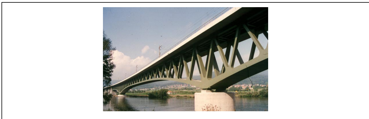
Figure 6 Railway bridge across river Main at Nantenbach
