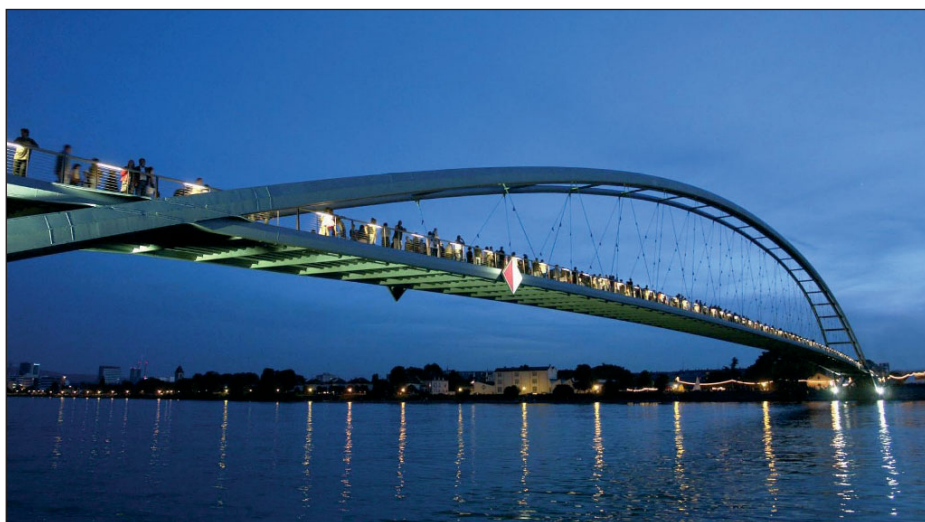
Fig. 11: Tri-Countries Bridge at night
