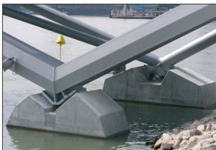
Fig. 6: Hünigen: fixed for longitudinal displacement
